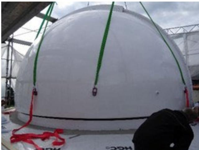
Figure 1.7: Installation of the new 6.15 m. slit-type dome for ZIMLAT.
