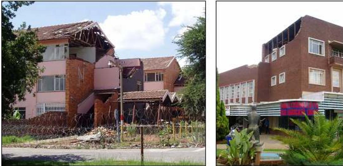
Figure 5. Damage in Stilfontein caused by the  $ML = 5.3$  tremor on 9 March 2005
