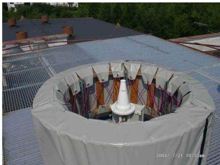
Fig. 4.10.1. Antenna A of the EGNOS RIMS station in Warsaw
